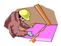
The three main types of loft insulation are blown insulation, blanket insulation and loose-fill insulation. Blanket and loose-fill insulation can be easily installed, but blown insulation must be installed by a specialist contractor.
